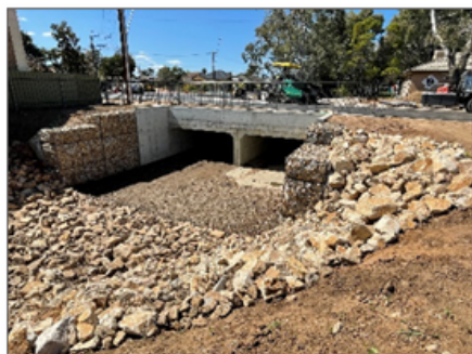
4 LBHC Daly Street Bridge
