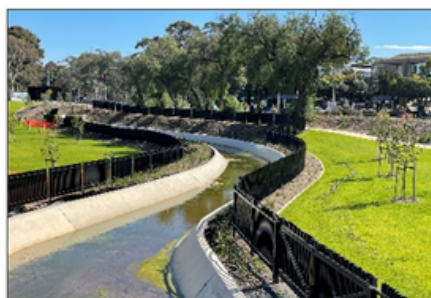
2 Glenside Detention Basin-Channel
